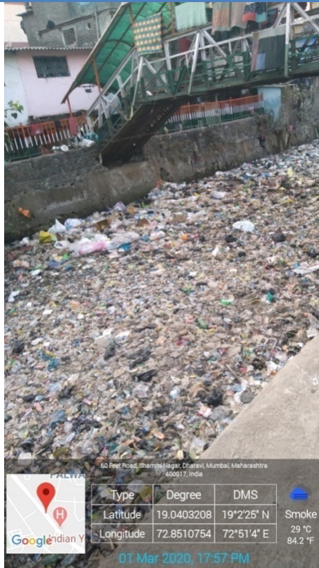
Plastic Dumped directly into Channel
