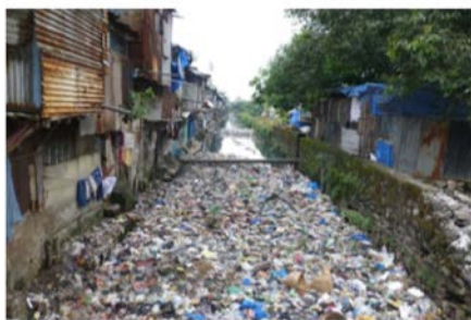
Photo indicates that thin Layer of Plastic Litter Clogged into drainage passing through slum areas
