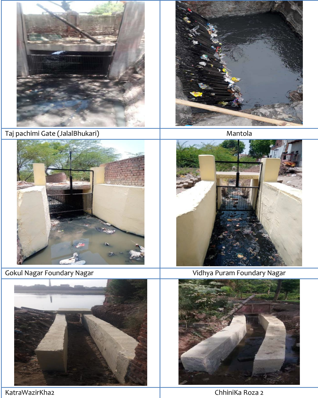
Figure A64: Drain Barrier in Agra
